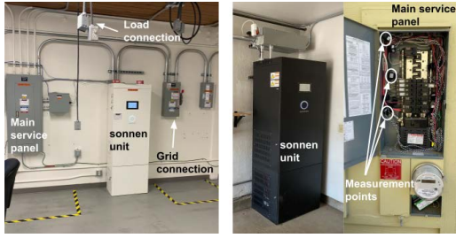
Figure 7: Photos of installed sonnen units. Left is the lab setup while right shows the home setups.
